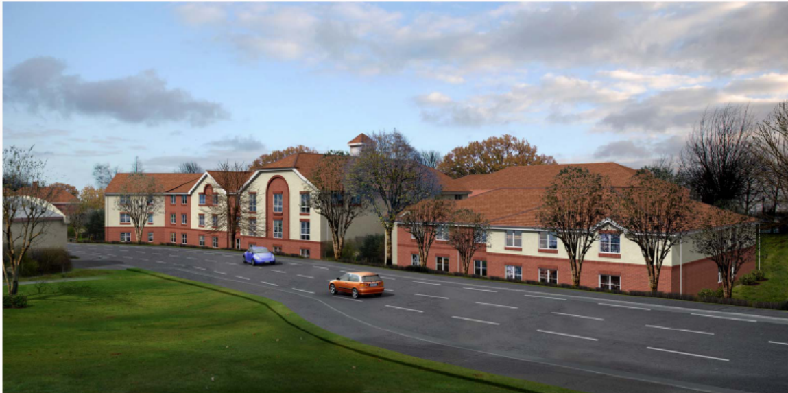
New Carehome Development - Nottingham Road, Nottingham
